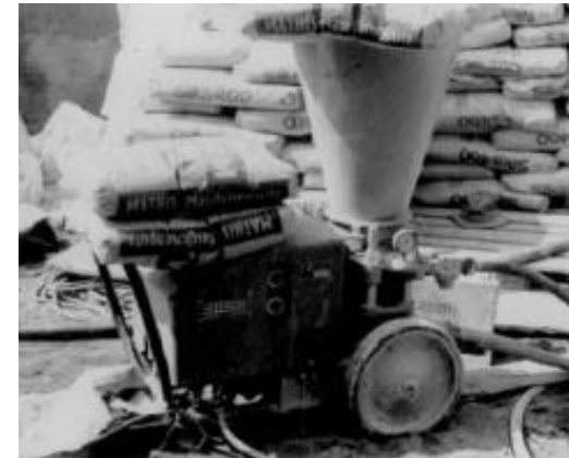
One of the first mortar mixers in action on a jobsite in Germany (1970)
