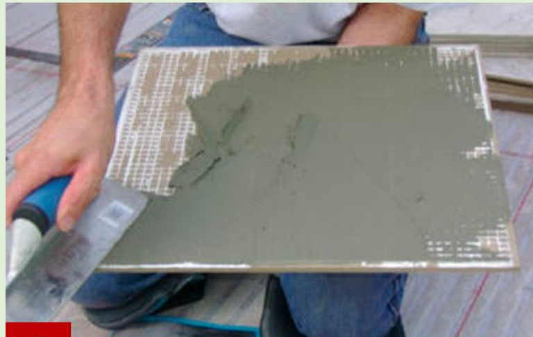
2 Apply a thin coat to tile back
