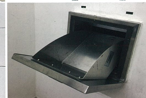
Gambar 6: Pneumatic Waste Conveying System (PWCS)
