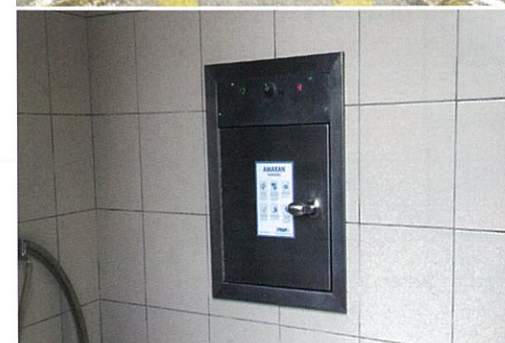
Gambar 6: Pneumatic Waste Conveying System (PWCS)
