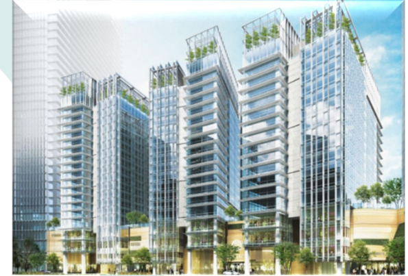
KL Eco City Boutique Office (The Pillar) SP Setia (a JV with DBKL)
