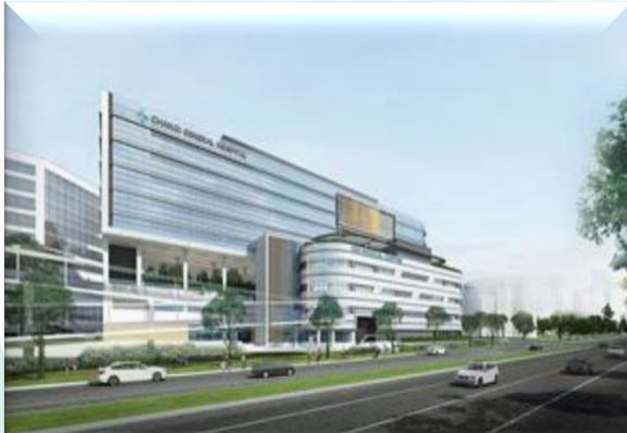
Changi General Hospital (Medical Centre) Singapore Ministry of Health
