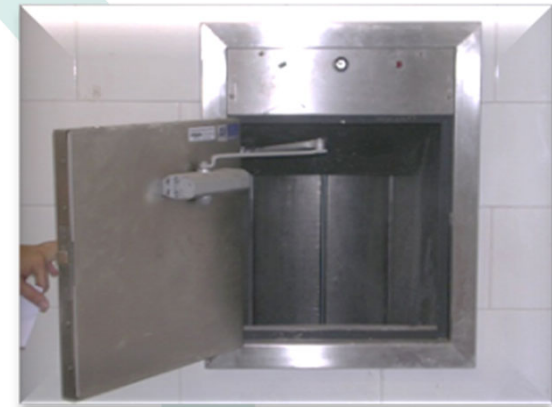
Full Vacuum Load Station's Swing Door & Inner Door
