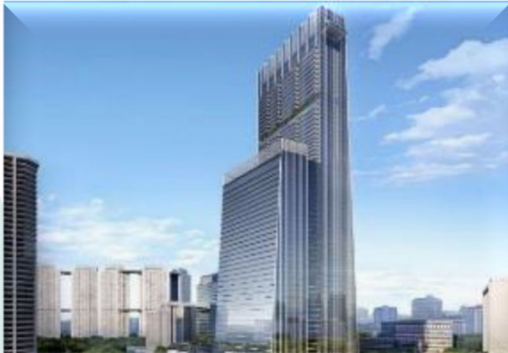
Wallich Residence (Tanjung Pagar Centre) Guocoland
