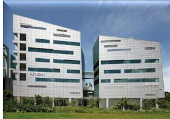
Biopolis Phase 3 Crescendas Bionix
