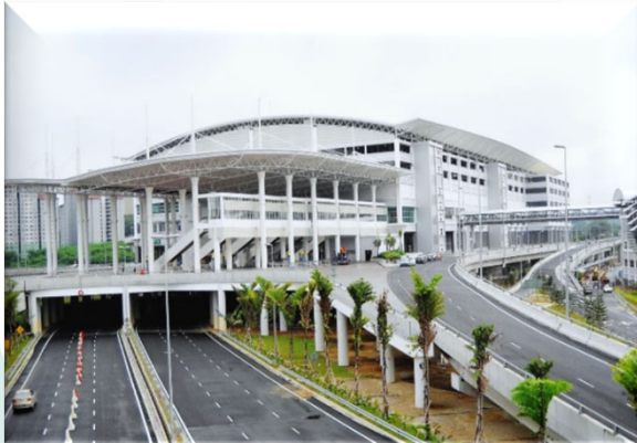
Integrated Transport Terminal- Southern Sector Ministry of Transport Malaysia
