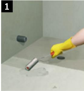
1 Surface preparation And/or screeding
