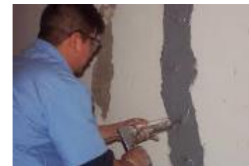
Crack fill works (interior & exterior)
