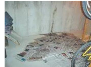
Rain leakage through cracks (inside)
