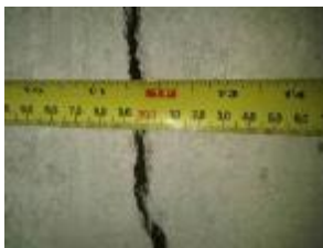
Wall crack on masonry wall (interior & exterior)
