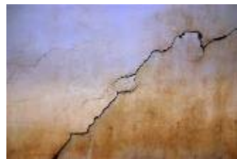
Wall crack on masonry wall (interior & exterior)
